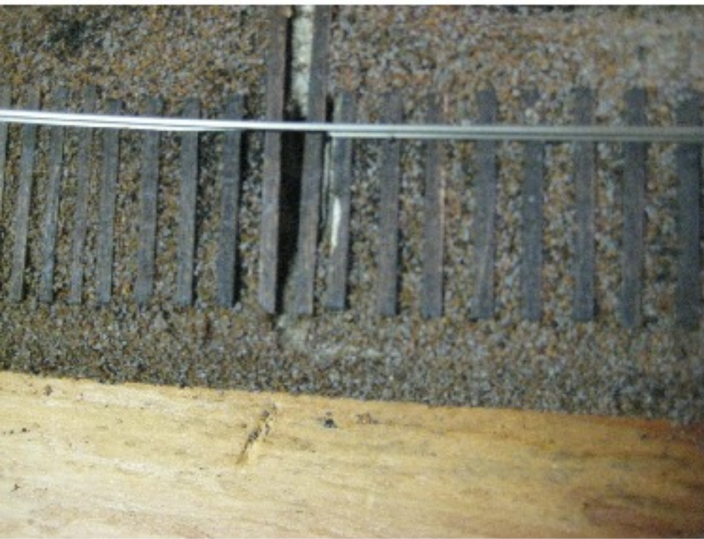
Stock rail w web removed
